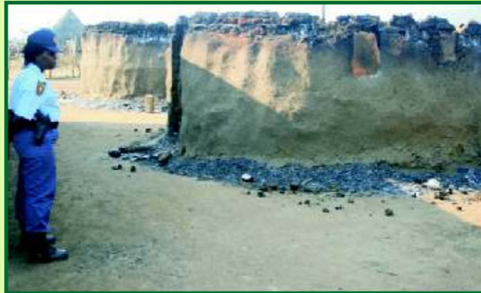
HOUSE ON FIRE: A Police officer stands next to the gutted hut at Mananga Village.
