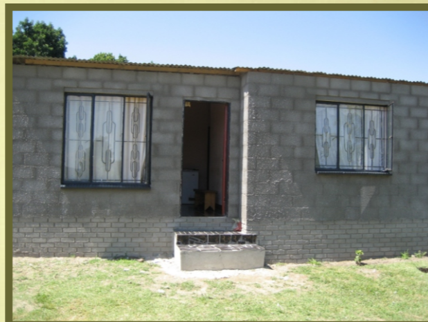
Ms. N. Hlabangane's new house completed within a month
